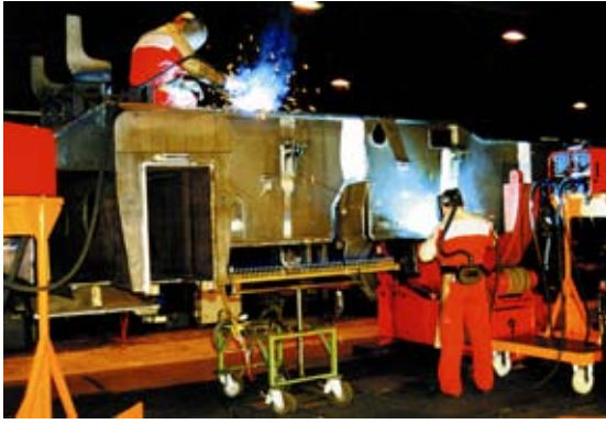
Figure 3 Welding fine-grained constructional steels in crane construction work
