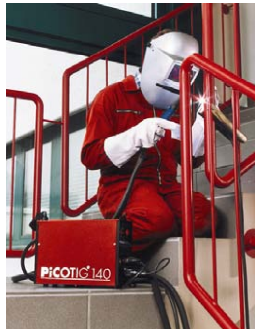
Figure 4 TIG welding on a beam
