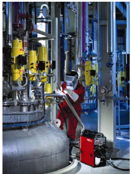
Figure 30 TRITON 260 DC, TIG welding on pipes
