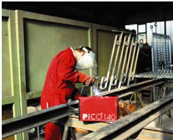
Figure 22 Use of MMA welding in beam construction
