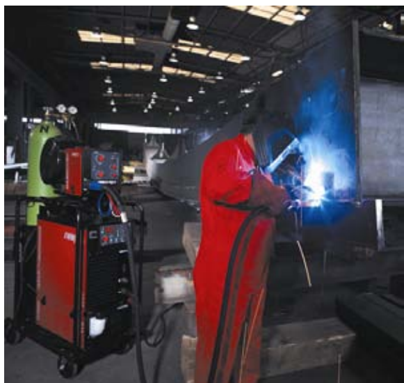
Figure 38 MAG welding on beams in steel construction work
