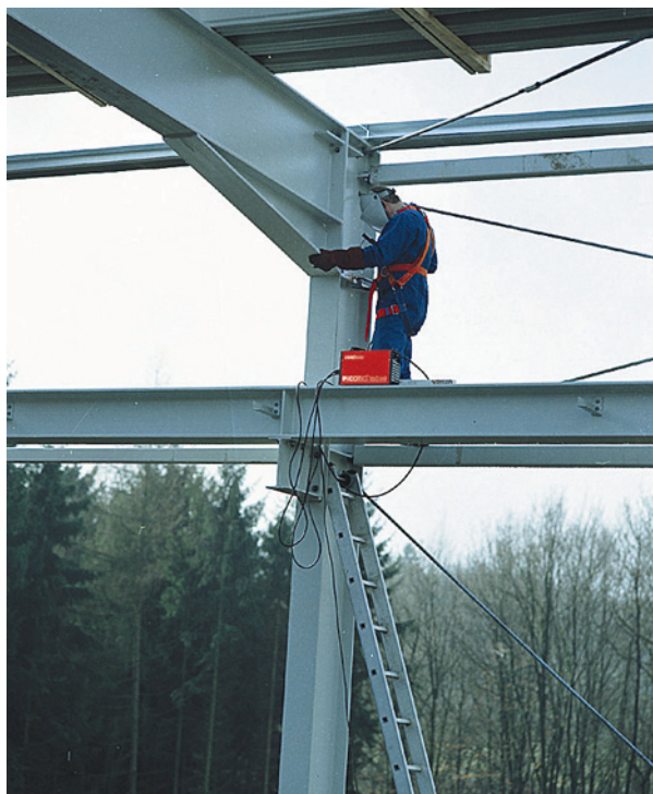
Figure 20 Use of inverter power source PICO 162 on a construction site
