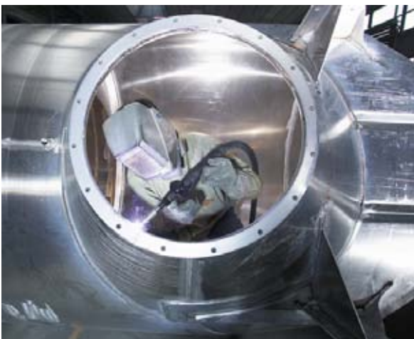
Figure 42 MIG welding used to manufacture tanks
