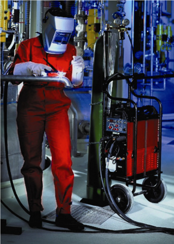
Figure 6 TIG welding work in the chemical industry
