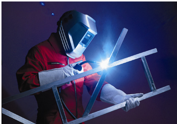
Figure 1 MAG welding in a workshop
