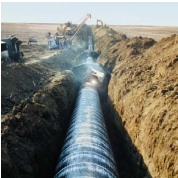
Figure 6 Welding in pipeline construction with cellulose electrodes
